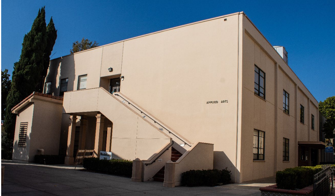
Photo 23 South elevation of the Applied Arts/Humanities Building; camera facing northwest
